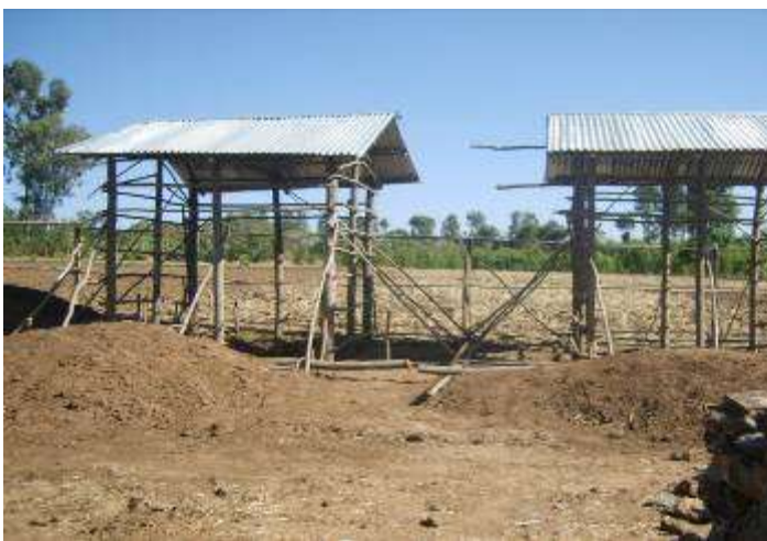
Construction of toilets at Chocha school
